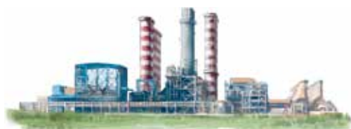
Newly-built refuse incineration power plant with a daily disposal capacity of 1,000 tons
